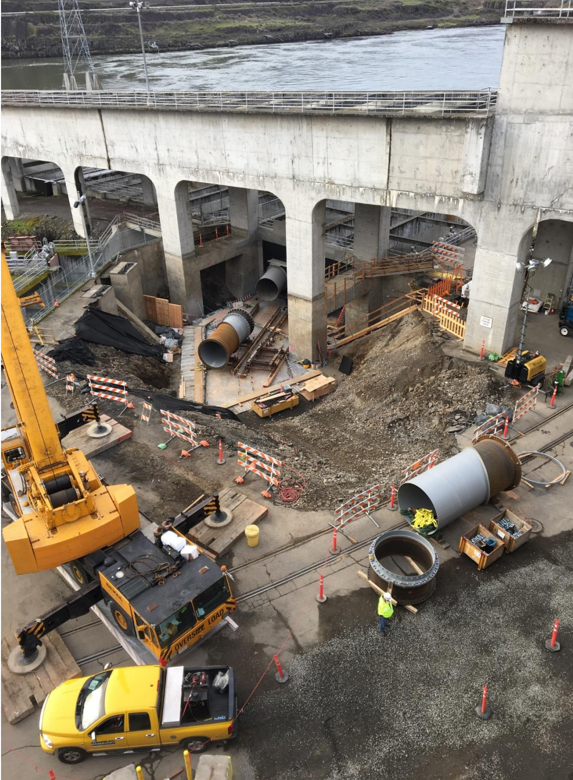
Installing AWS 7' pipe sections.
